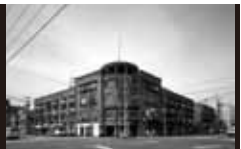
Dojunkai Building [1926-1934] YS Dojunkai Building Department
